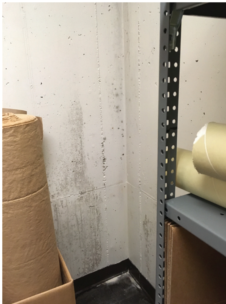
A dead air pocket of in this corner of a basement corner trapped moisture and caused black mold to grow on the walls.
